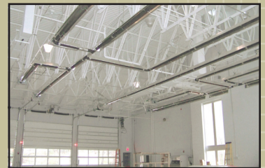
Fire Station Apparatus Bays
